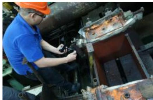
**Gambar 7.** Pemasangan compact transmitter
